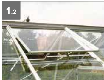
1.2 Window Exterior view
