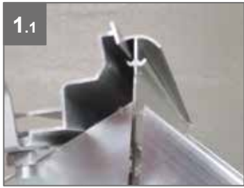
1.1 Installing the window on roof ridge through sliding
