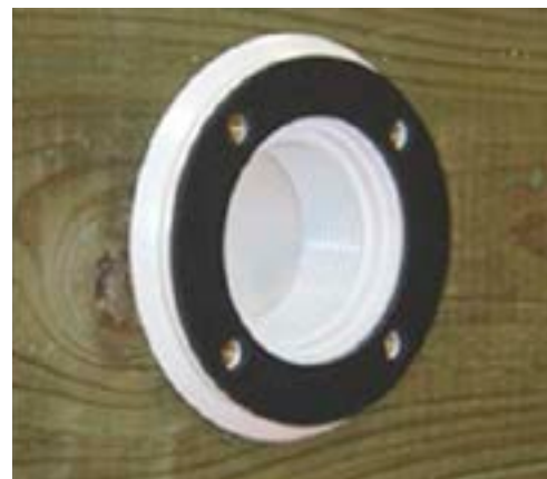
Figure 19 – Pose du joint
