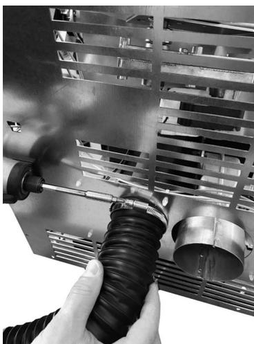
*Fig. 13 - Raccordement air comburant*
