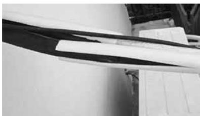
10. At last, use the tape to wrap the refrigerant pipe and connecting cable together.
